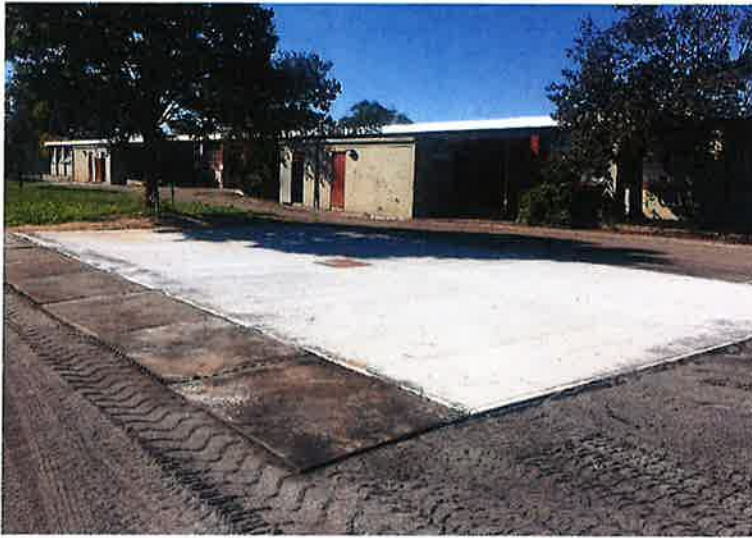
Photograph 3 – New wash pad constructed between barns 12 and 12A
