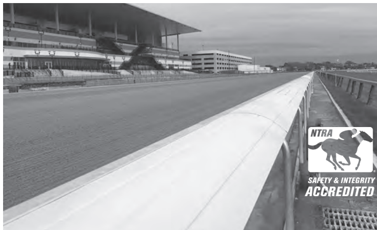
The new safety rail on the Aqueduct main track, the first of its kind at a NYRA track and one of several safety-enhancing capital improvements NYRA has undertaken since 2013.
